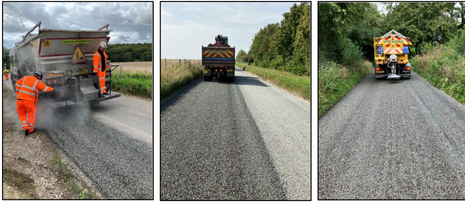
An extensive programme of surface dressing helps seal and protects the county's rural roads, and improves skid resistance.
