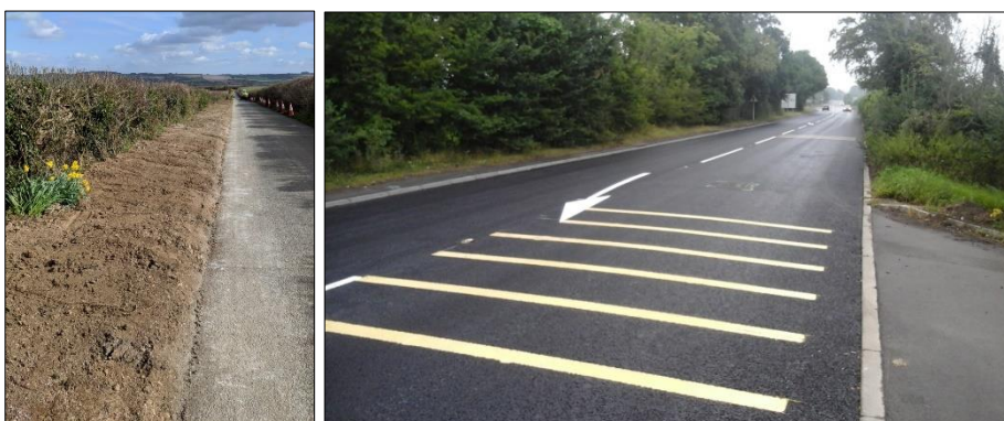
Verge, drainage repairs, and alterations to lane markings may be included in road maintenance schemes.
