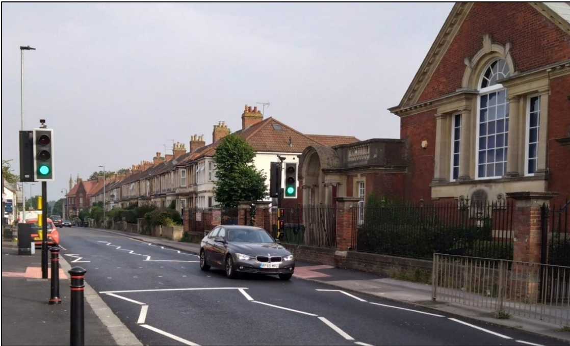
Newtown Trowbridge Puffin crossing replacing a previous zebra crossing
